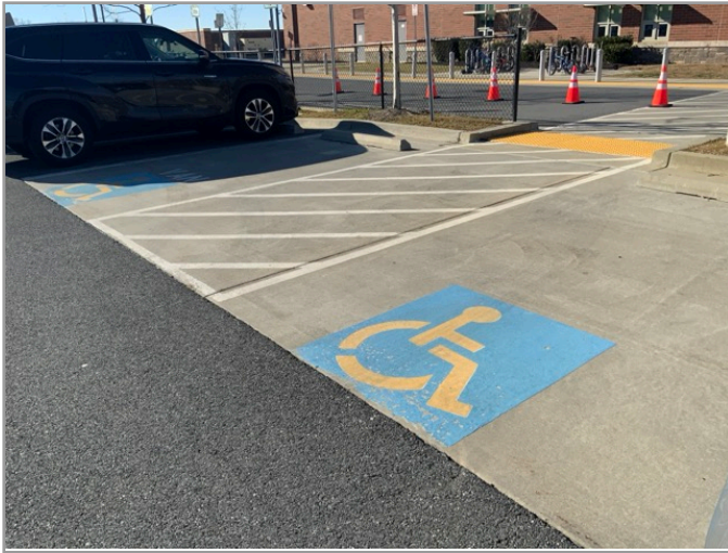
OVERVIEW OF ACCESSIBLE PARKING AREA
