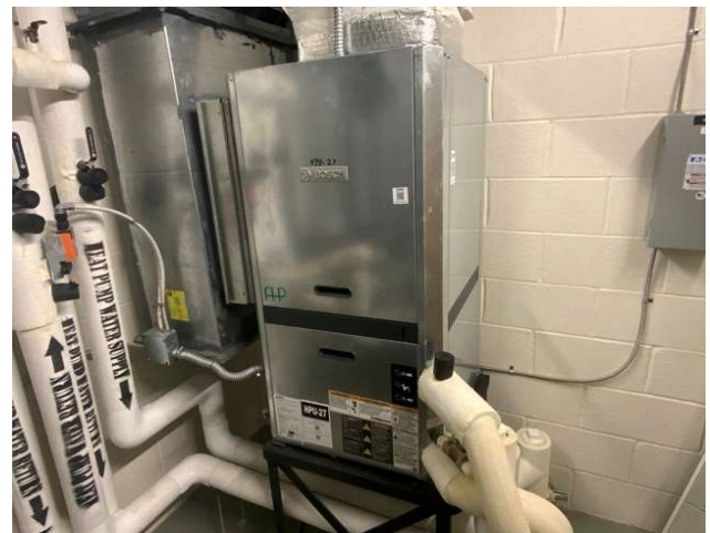
10 - TYPICAL WATER SOURCE HEAT PUMP
